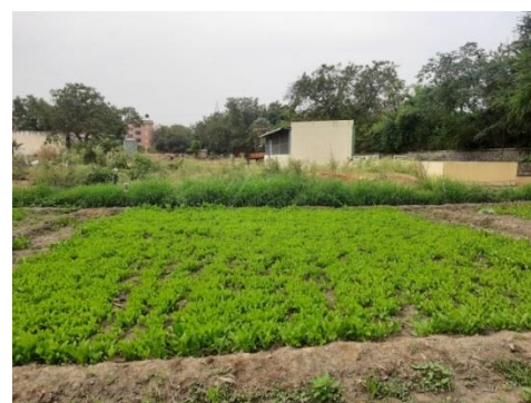
STP double filter for irrigation
